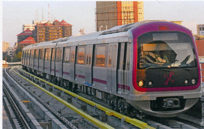
The most modern driverless metro coaches result in maximum utilisation of the available network.
