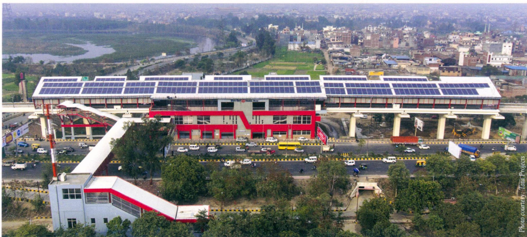
Energy-efficient technologies such as solar panels on-site/off-site installations make metro systems more eco-friendly.
