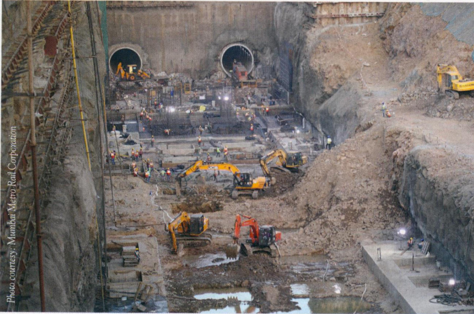
TBMs, excavators, road headers, hydras, cranes, gantries, piling rigs, batching plants, transit mixers and boom placers, is being used in metro projects.
